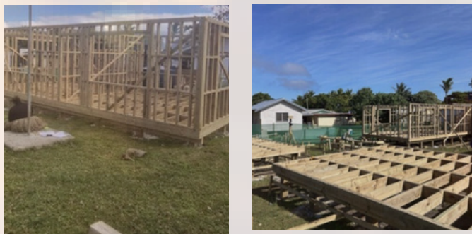
Figure 5&6 : Timber Frame Wall for Classroom and Wash Facility
